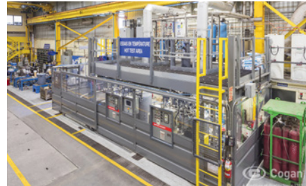
Secure storage & space solutions to protect assets
