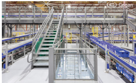
AMR's (automated mobile robots), conveyor systems & integration
